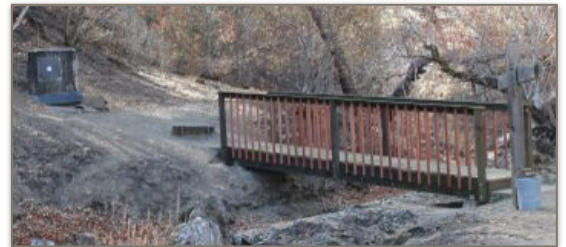
The bridge to target 3 that Pat and his crew rebuilt.
